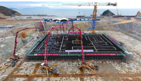
The CFR-600 construction Source: www.neimagazine.com
