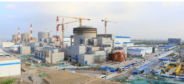
The Tianwan NPP construction
